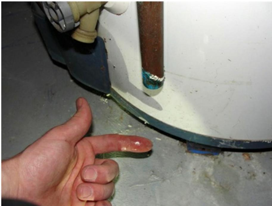
1. Initially ensure it is the water heater that the leaking water is originating from.
